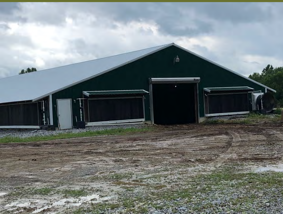
One of two mega broiler houses located on Brockman's property.
