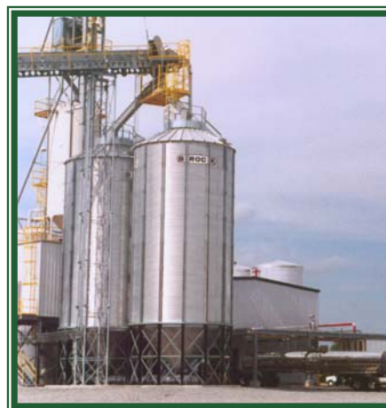
Commonwealth Agri-Energy Kentucky's first ethanol plant.
